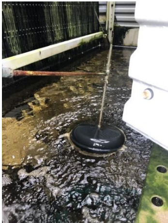
Tower Sump with Significant Biological Fouling
