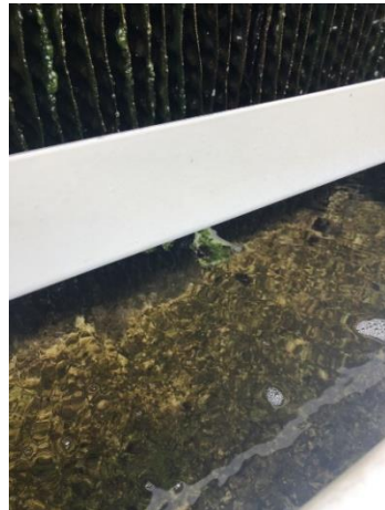
Tower Sump with Significant Biological Fouling
