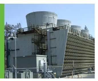
You will also need to clean and treat the water for your cooling tower if you have a new system. Shipping and installation of the tower components could cause damage or leave materials (https://www.chardonlabs.com/cooling-towers/#link7) on the surfaces that lead to corrosion. Cleaning removes these from the surfaces and prepares the tower for the treated water.
